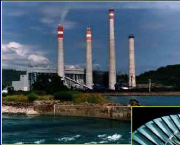
Steam Power Plants
