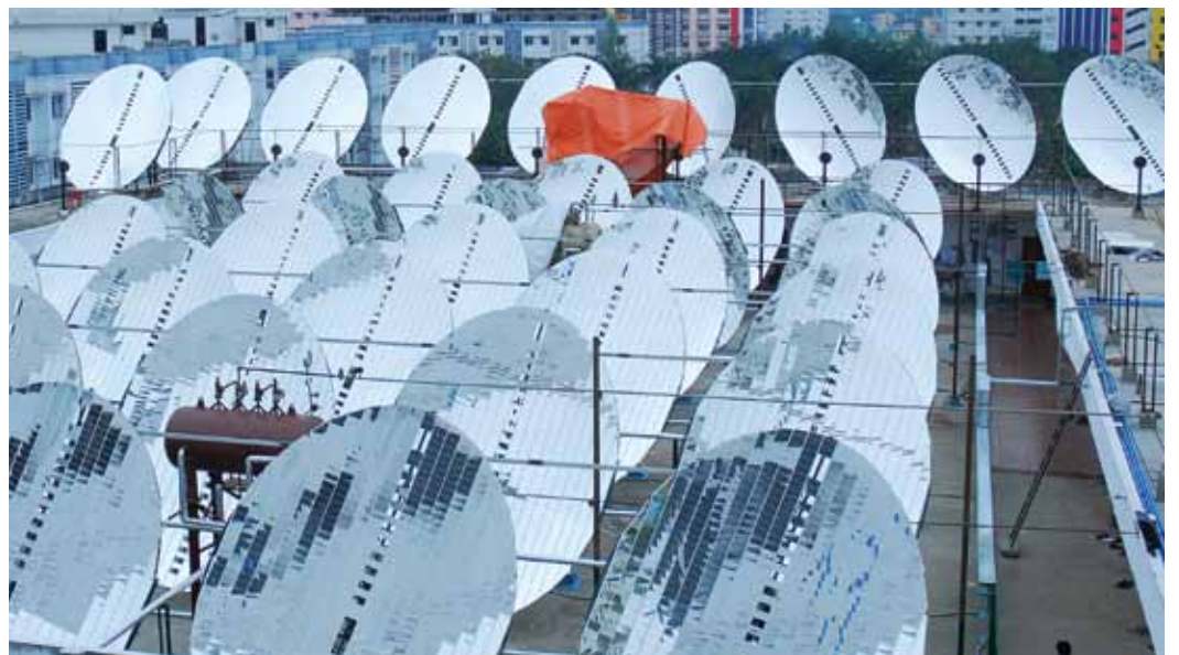
Solar panels for heating water
