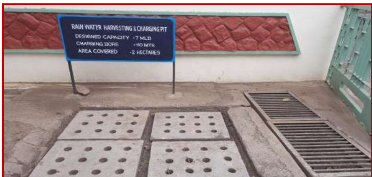
Fig.6: Sample Rain Water Harvesting (RWH): Storage and Name Board Representation
