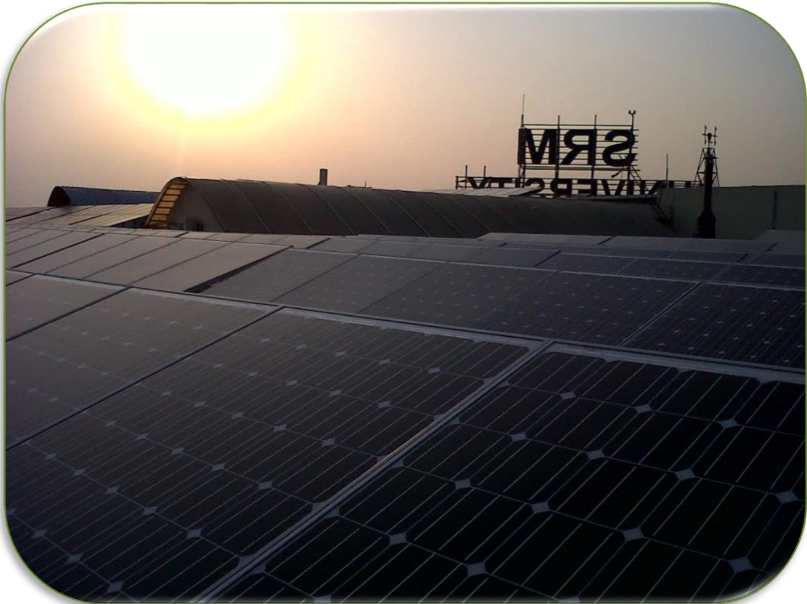
Figure 2 : 100 kW solar panel installed at University Building
