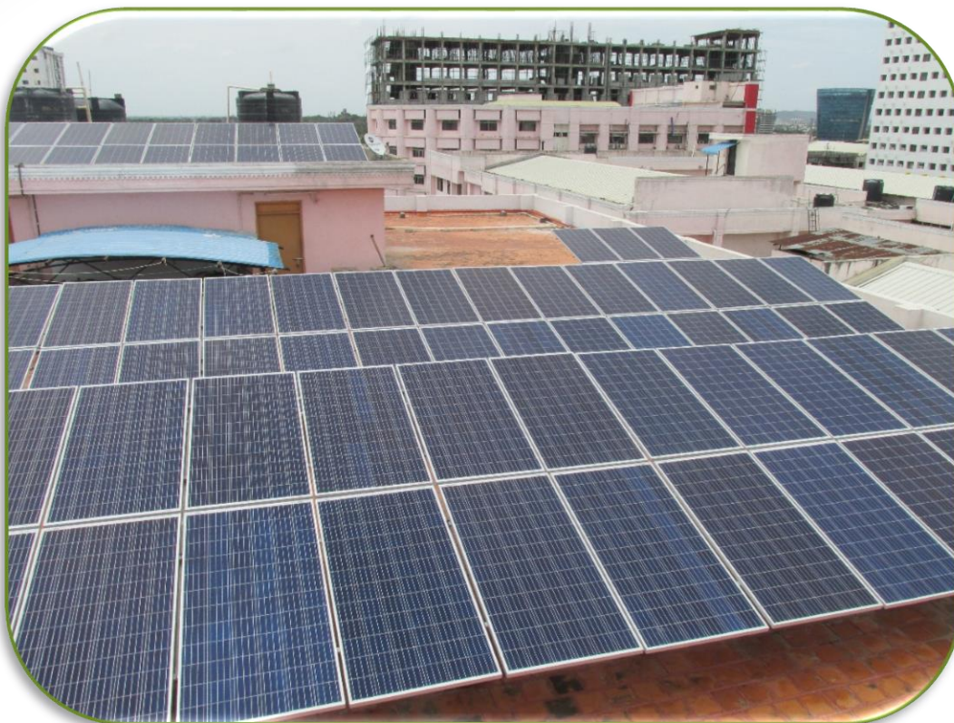
Figure 3 : 55 kW solar panel at Basic Engineering Block
