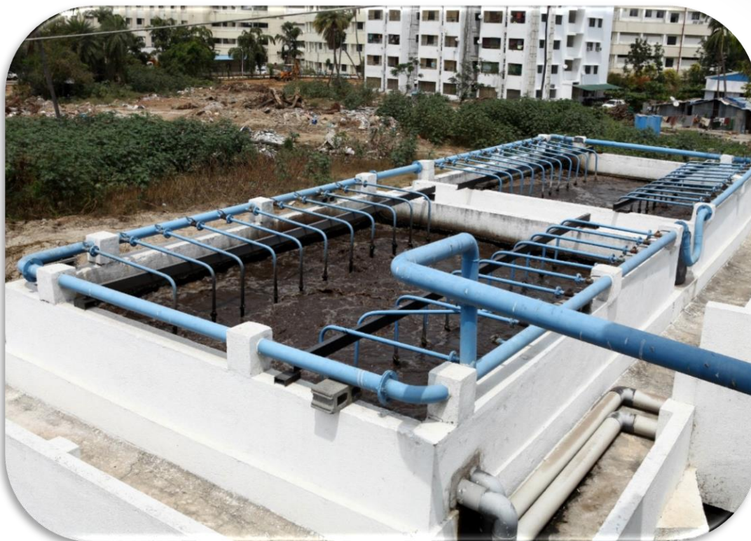
Figure 37: Clarifier tank in wastewater treatment process
